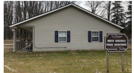
Safetyville Building 35753 Bainbridge Rd. North Ridgeville, OH 44039 Alternate Drop off & Pick Up
